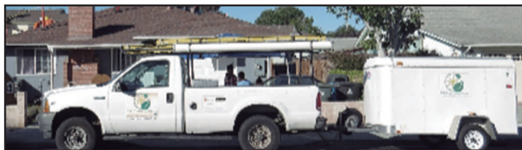
The truck carries all of the hardware that is required for the solar installation on Chris and Lea Martinez' house.
