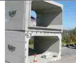
Photo courtesy Sean Charpentier A photo of one of East Palo Alto's new storm drain systems
