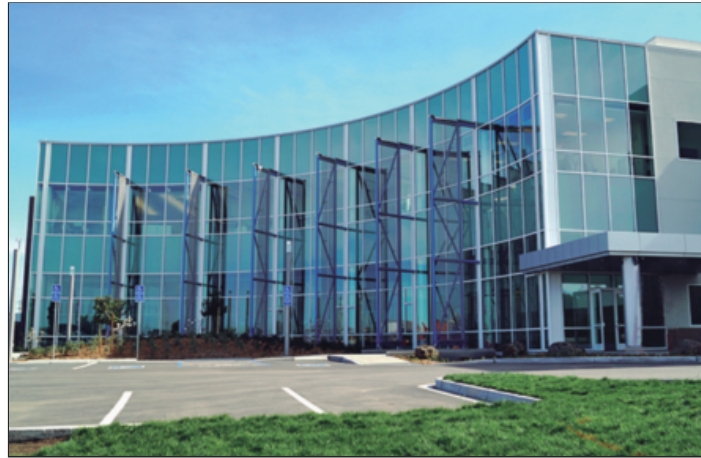
Photo courtesy of the County of San Mateo This state-of-the-art jail was opened at 1300 Maple Street in Redwood City on March 1, 2016. It's design is said to "optimize staff and occupant health through access to daylight, fresh air and radiant flooring and its steel walls allow for [the] greatest security with [the] smallest footprint. It also has 14 original art pieces.
