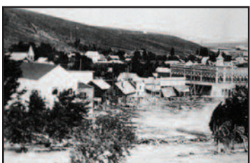
Photo shows houses underwater during flooding
