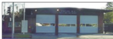
Photo courtesy of the Menlo Park Fire District website This photo shows the East Palo Alto firehouse that is under construction.
